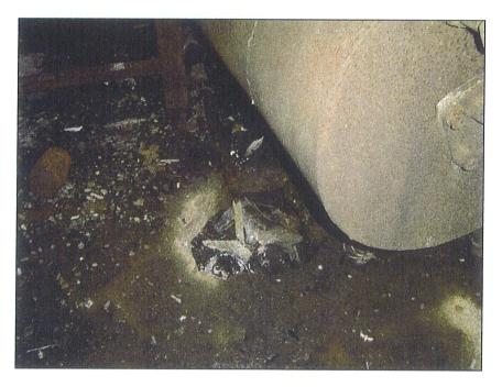
Photograph 20: View of the hole in the concrete floor of the boiler room.
