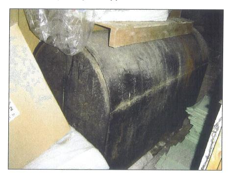
**Photograph 2:** View of the 275-gallon aboveground storage tank (AST) in the utility closet.
