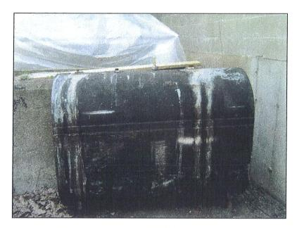
Photograph 15: View of the 275-gallon AST with staining located at the N side of the loading dock. The tank is not connected to building or currently used.
