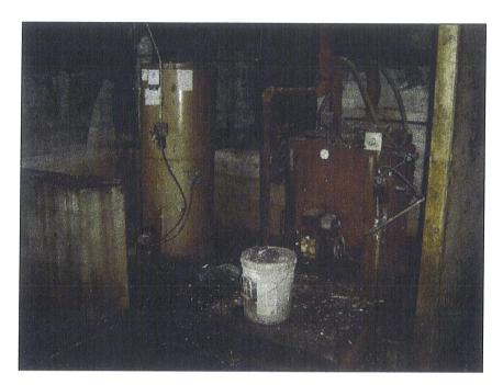
Photograph 19: View of the portions of a former boiler and oil-fired hot water heater inside boiler room.
