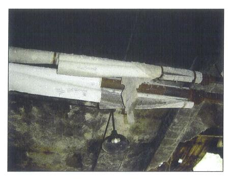
Photograph 21: View of the suspect asbestos-containing building materials (pipe insulation) in the former boiler room (poor condition).
