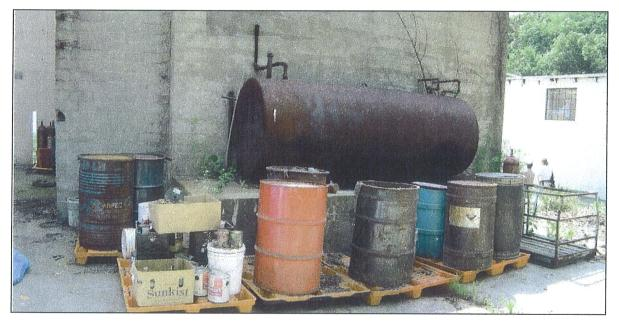
Photograph 16: View of the leaking 1,000-gallon #2 fuel oil AST located on a concrete platform. Tank is not active but was used when central boiler was active. View of the drums of various content and origin stored on fork truck pallets (orange) N of old boiler room.
